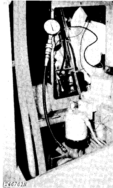
Fig. 2-Oil Pressure Test Connection Point
